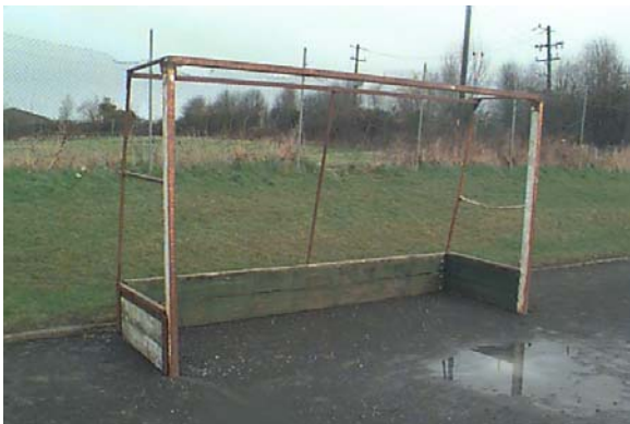
Hockey goal. Frame with rectangular section having sharp edges. Frame rusty. Upright buried directly in concrete - should have ground anchors.
