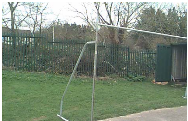
Portable GAA goal - no anchoring provided. When upper posts in place the goal frame is unstable.
