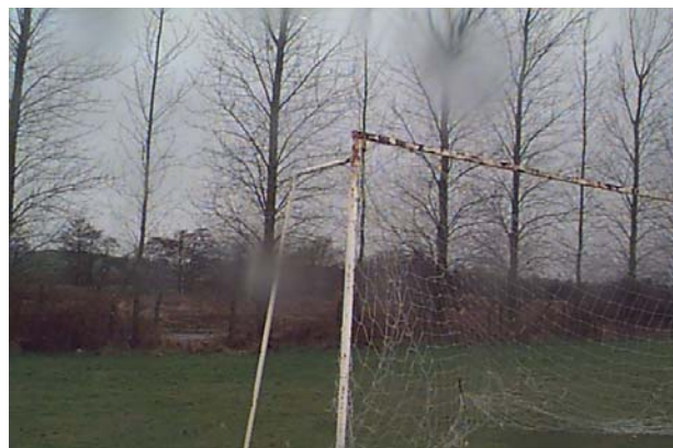
Soccer goal frame with square section having sharp edges.
